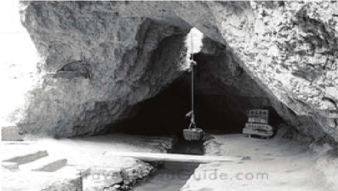
**Fig.2.6 :**Construction d'un karez dans Turpan, Xinjiang, Chine\_ Qingwei Sun, Tao Wang, Iwao Kobori, and Luohui Liang\_2006
