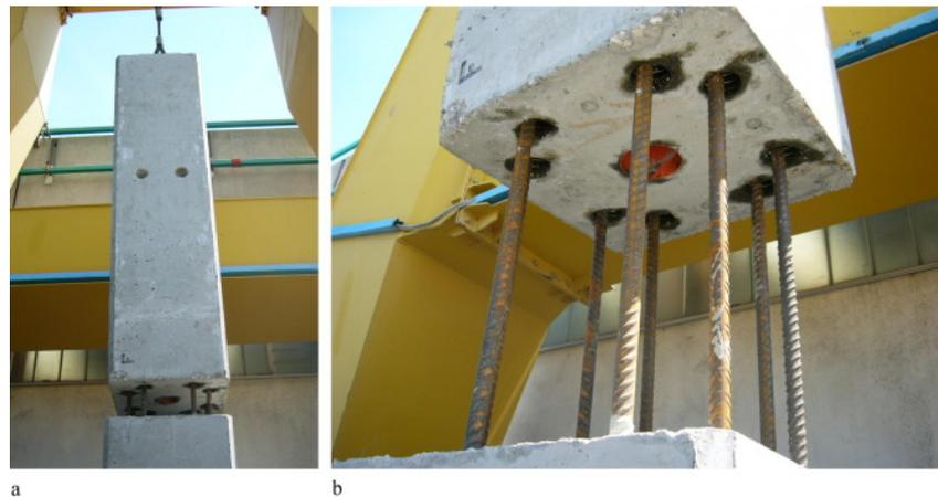
Figure 1.9 – Connexion poteau-poteau
