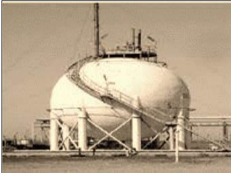
Figure 1.7: Ballon de stockage
