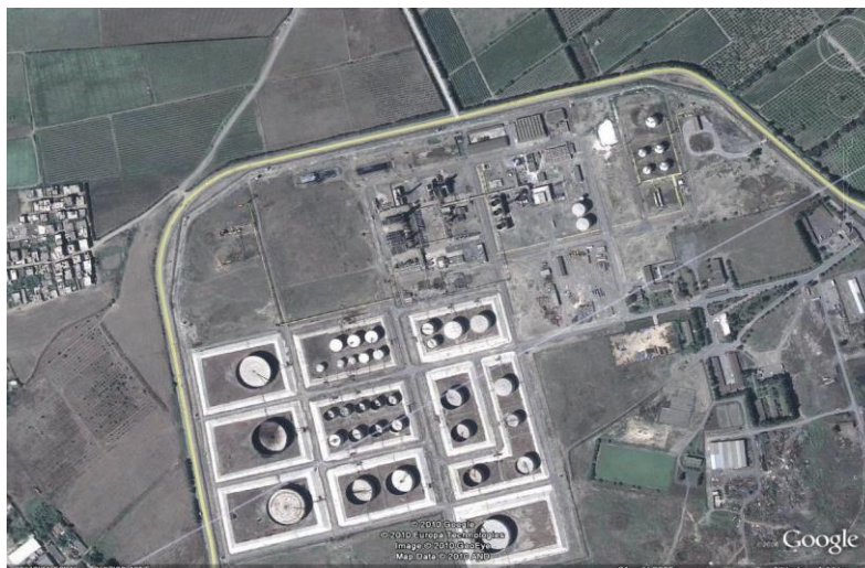
Figure 1.8- Raffinerie Sidi -Arcine- Alger
