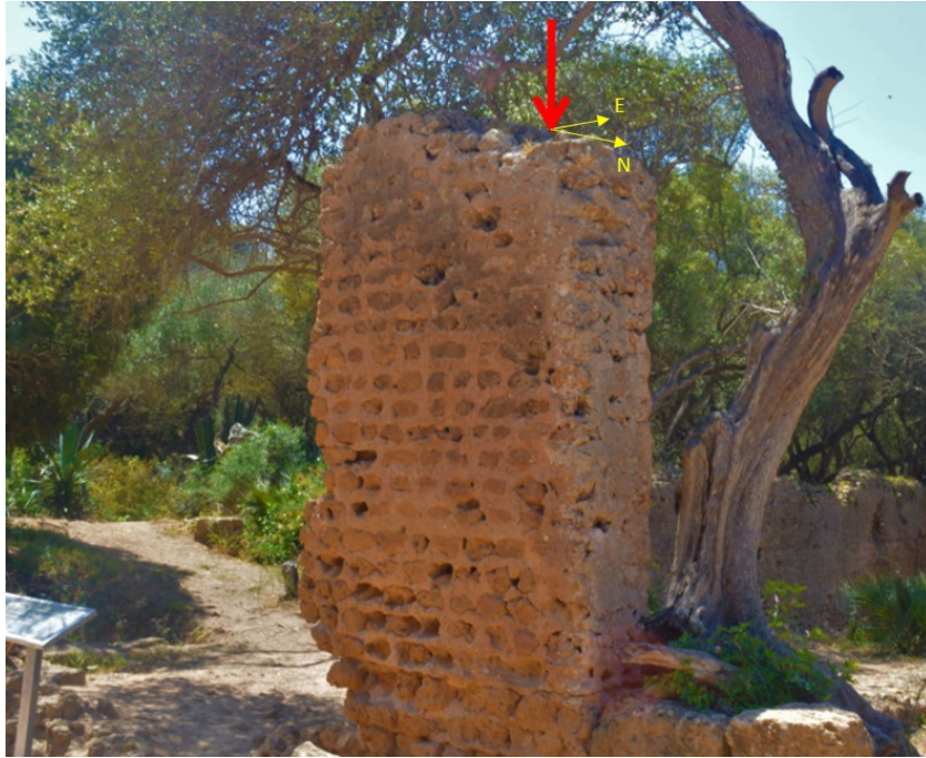
Figure 4.7: Measurement Points on the wall.
