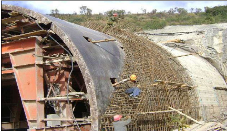
Figure 2.16 : coffrage armé M3 (cosider tp) [19]
