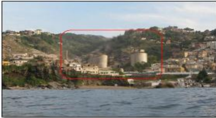
Figure I.1: Cimenterie de Rais Hamidou
