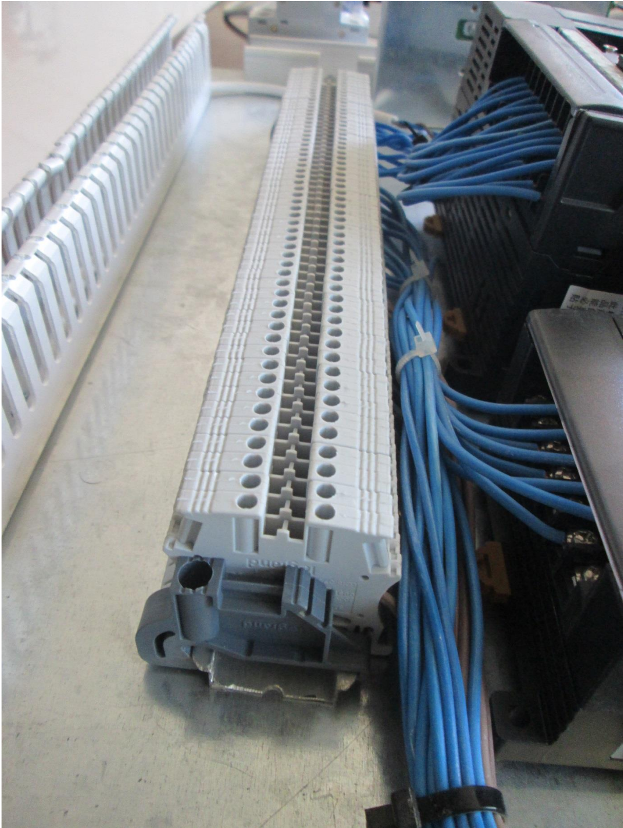
Figure 1.58: Legrand Viking 3 terminal blocks with end-stops
