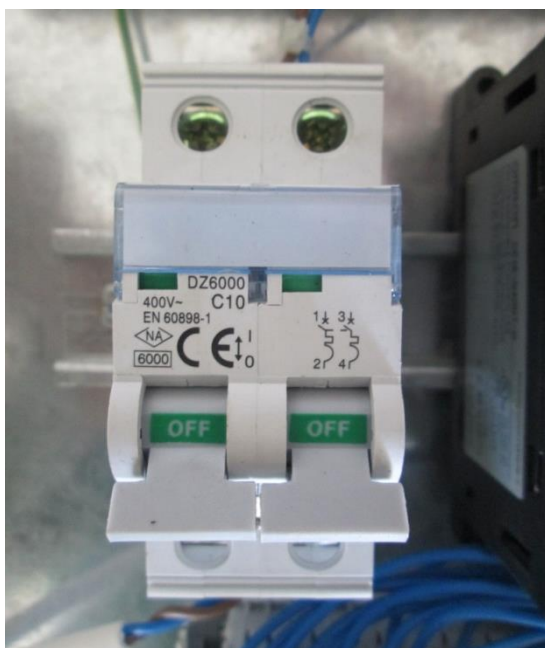
Figure 1.44: BMS DZ6000 C10 circuit breaker.
