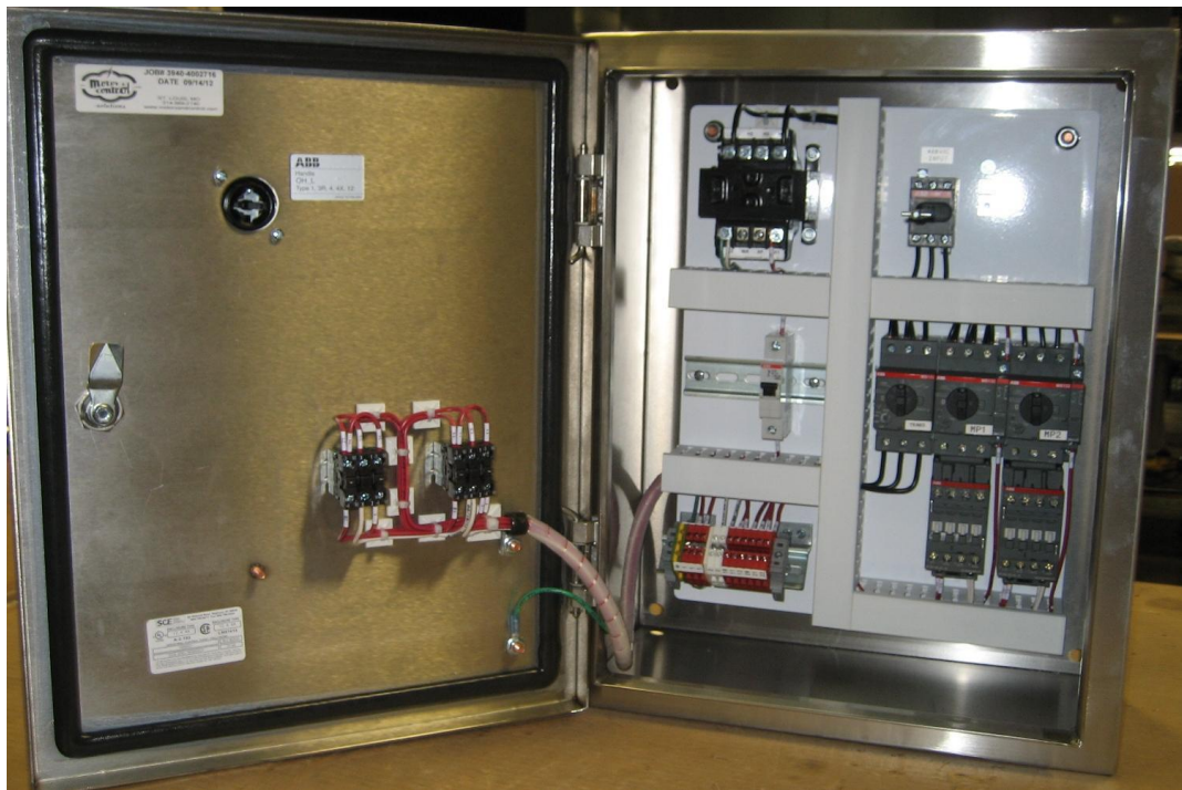
Figure 1.73: Stainless steel enclosure.
