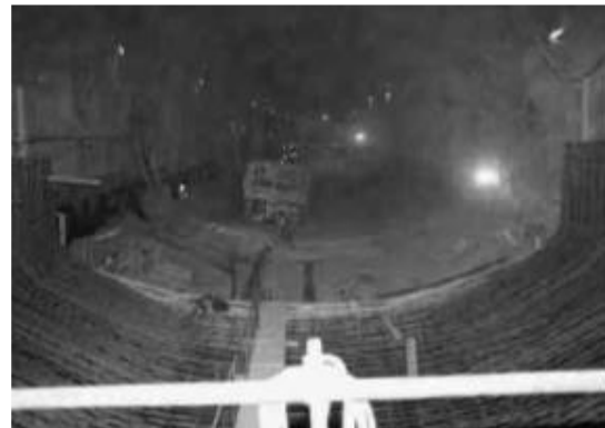
Figure III.10 : Armatures radier
