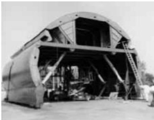
Figure III.9 : Coffrage de tunnel
