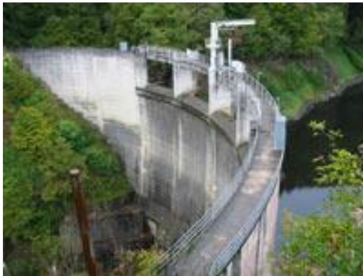
Figure II.4 : Barrage de Luzège[11]
