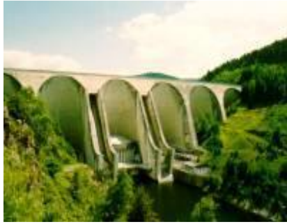
Figure II.6 : Barrage de Grandval
