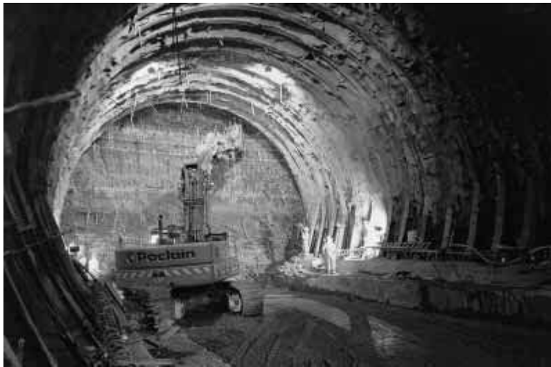
Figure III-1: creusement a pleine section.
