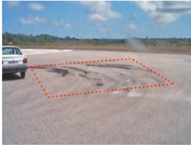
Figure II.11 : Fissure parabolique
