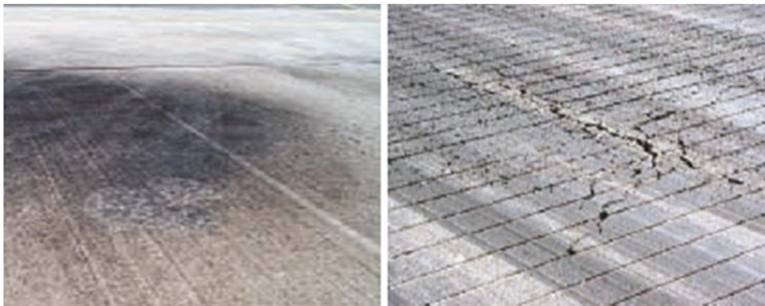
Figure II.21 : Ecaillage/Faïençage
