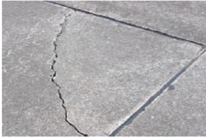
Figure II.16 : Fissure d'angle
