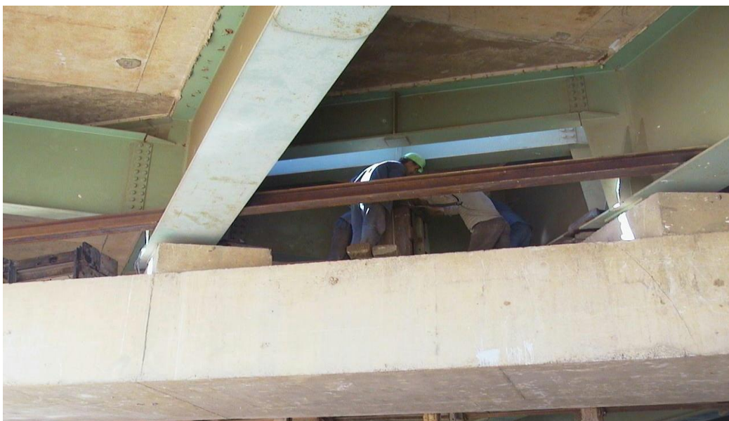
Figure V.18 Rigidification le tablier
