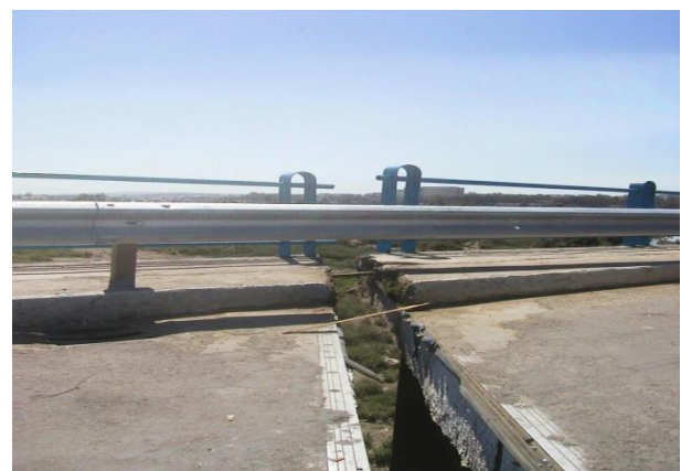
Figure V.7 Endommagement des joints de chaussée
