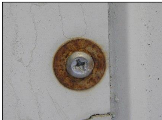
Figure I.15 Corrosion galvanique [23].
