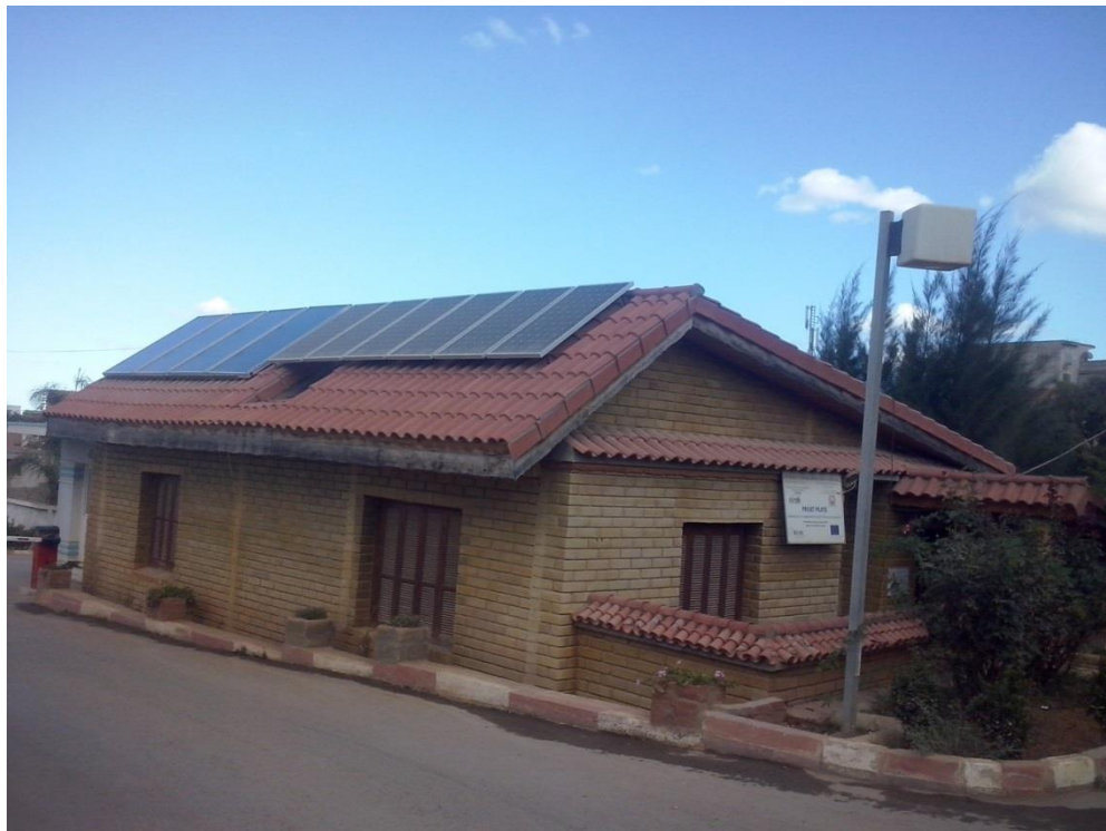
Fig 5.1 General view of the housing studied (Souidania, Algiers) and the photovoltaic array installed on the roof.
