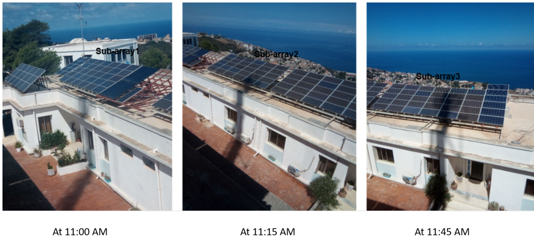
Figure 4.8: Position of the shadow on the three sub-array 1.2.3 on the day of 04/09/2020
