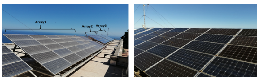
Figure 4.33: Dirty sub-array1 and cleaned sub-array2,3
