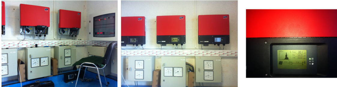
Figure 3.4: Sunny boy, 3000TLST-21 inverter
