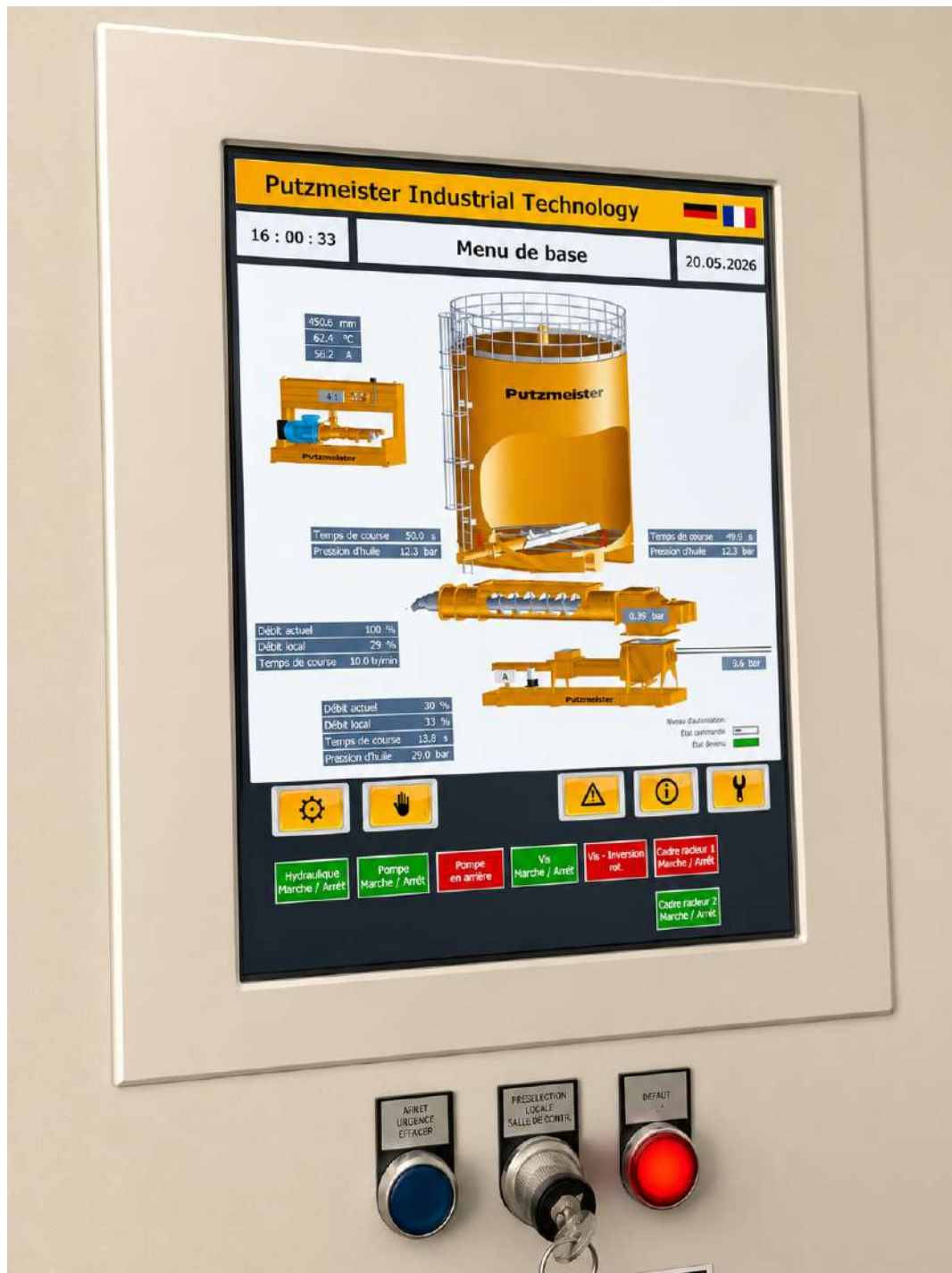
Figure 3.2. The Putzmeister injection-pump control screen at the Sludge Treatment Station.
