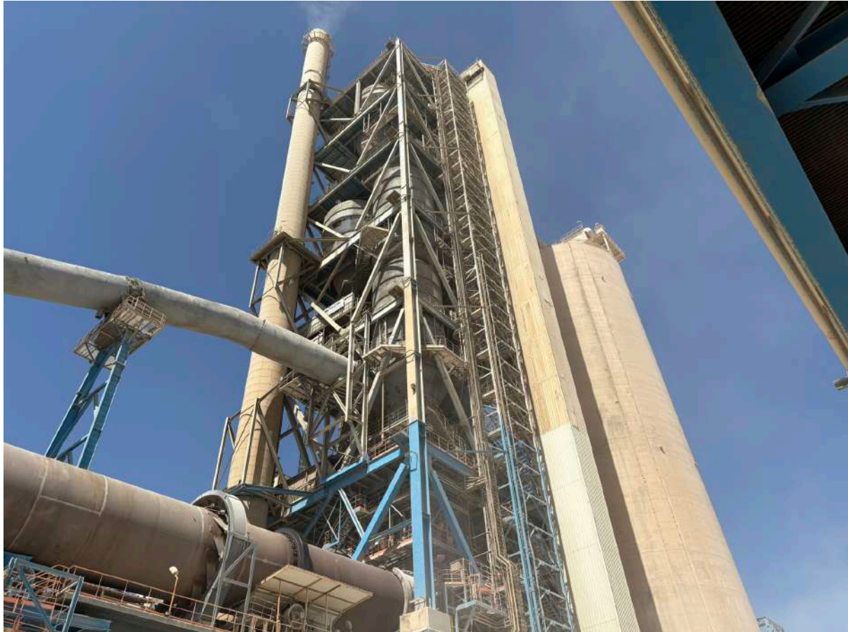
Figure 1.4. The five-stage preheater and calciner tower at Holcim El-Djazair – Oggaz.
