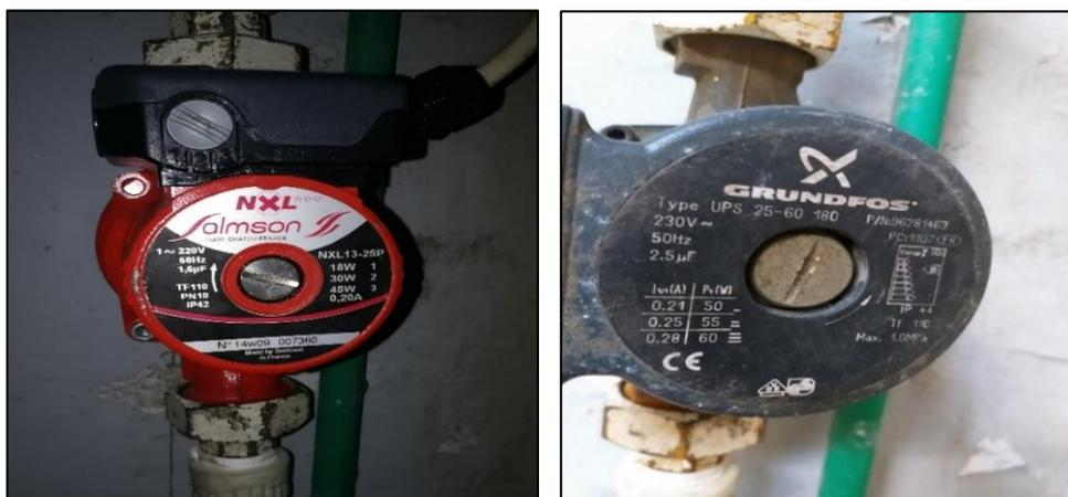
Figure III- 7: Circulating pumps.
