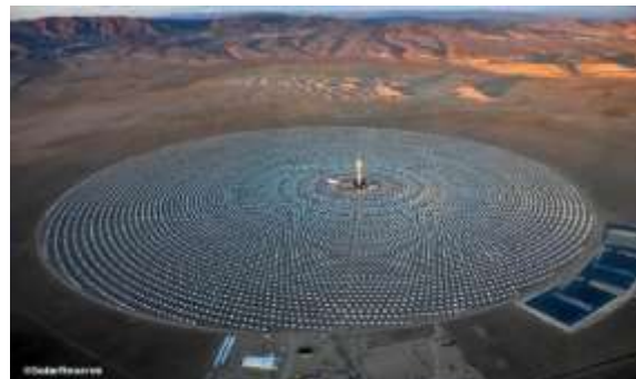
Crescent Dunes Solar Energy Project
