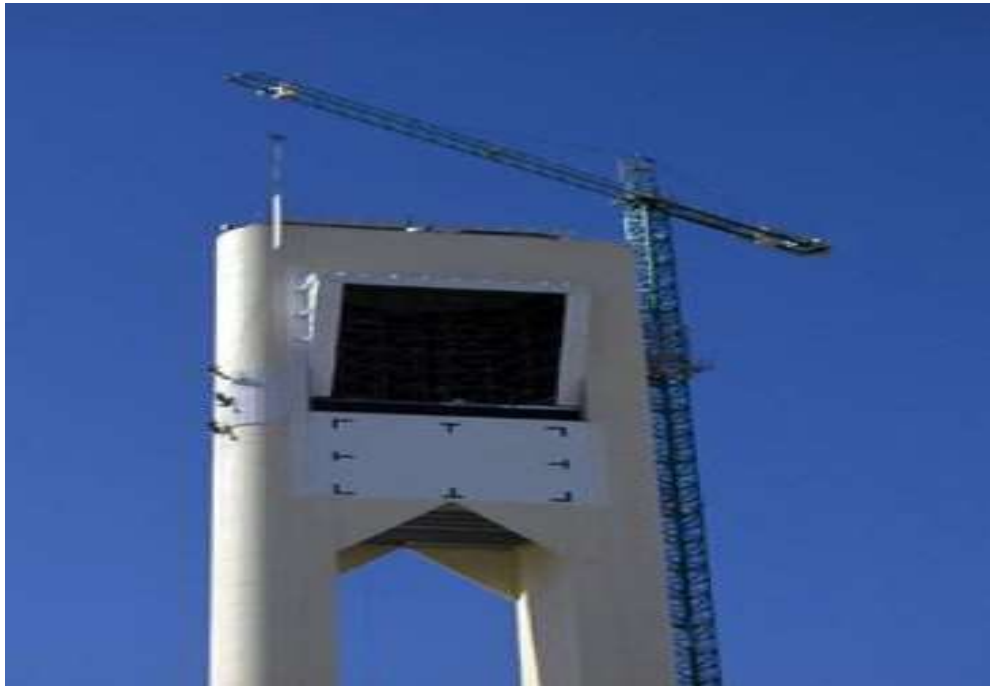
Figure 1.16. Cavity Receiver used in PS-10 [57]
