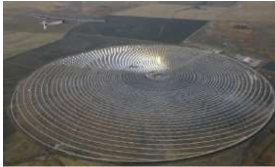
Gema solar thermo solar plant
