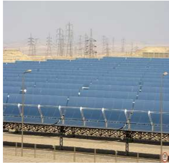
Figure 1.3.b. 140 MW ISCC Kuraymat, Egypt [39]
