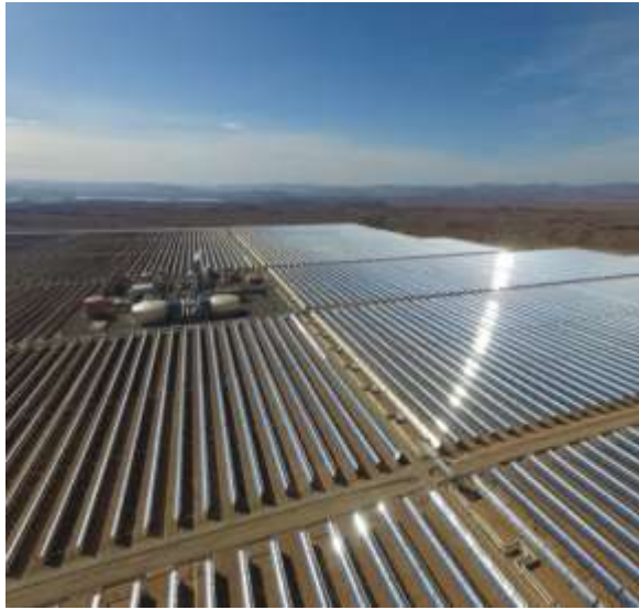
Figure 1.3.a. 160 MW NOORO I CSP, Morocco [38]
