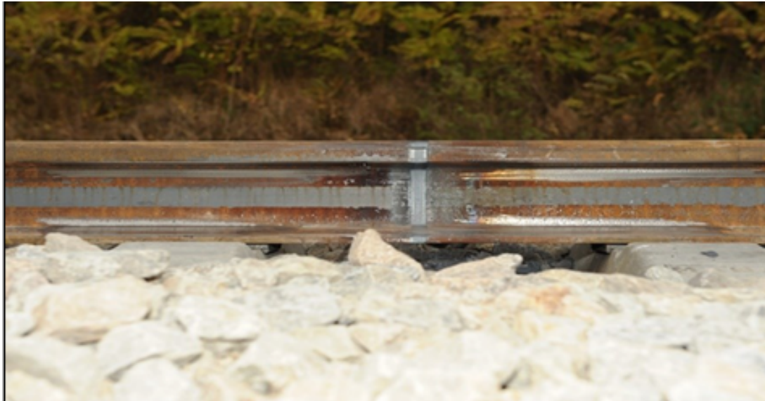
FIGURE 5.2 – Rails soudées.
