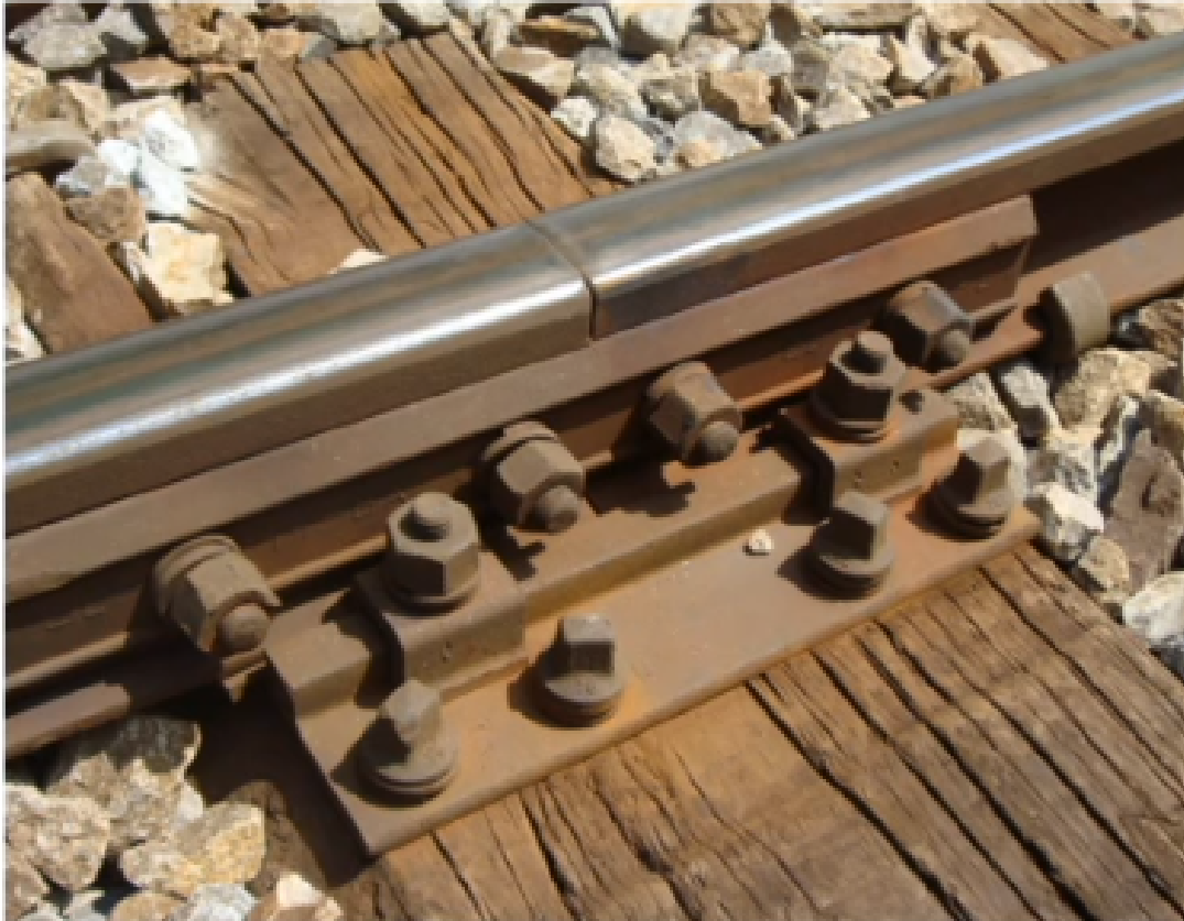
FIGURE 5.1 – Fish Plate Joint.
