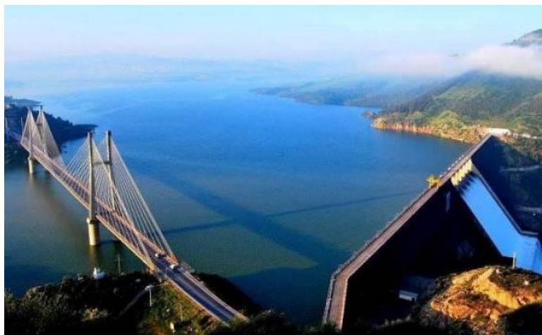
Figure 2 : Barrage de Beni Haroun, Mila
