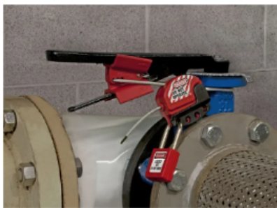
Butterfly valve lockout
