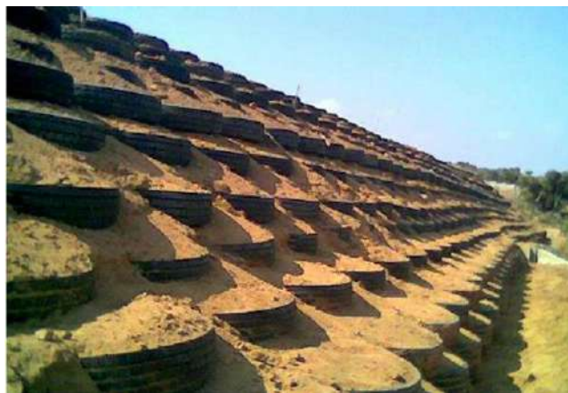
FIGURE 1.6 – Chantier Pneusol à Bou-smail.
