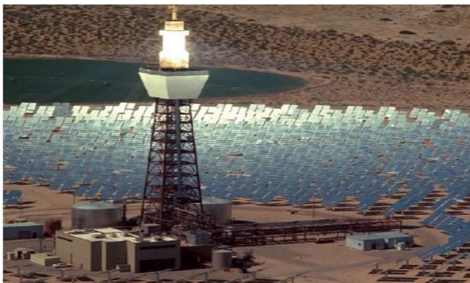
Figure I-14 : Centrale à Tour (Solar Two, California (Daggett)) [25]
