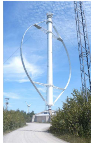
(b) Éole turbine 2 in Cap-Chat, Québec, Canada rotor diameter: 64 m, rotor height: 96 m, total height: 110 m, rated power: 3.8 M.
