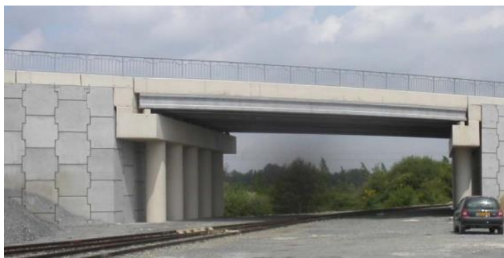
Figure 1.6: Pont de Saint-Pierre-la-Cour (France, 2001)
