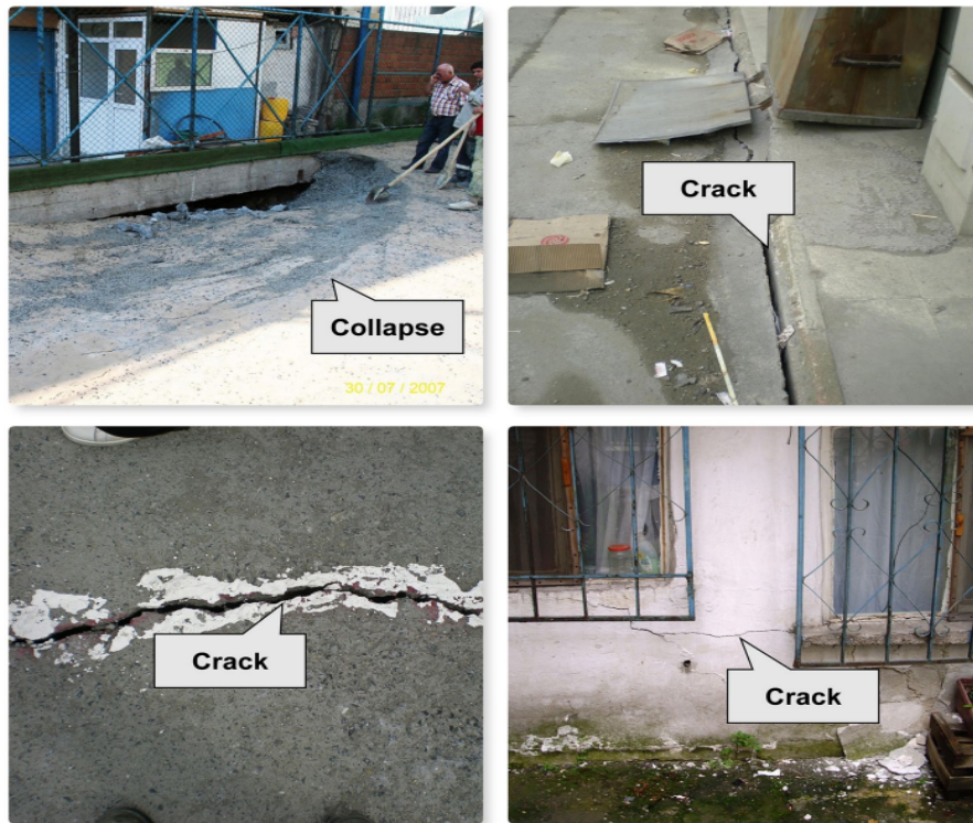
Figure 0.2: Damage caused by twin tunnel excavations along the Esenler–Başakşehir subway line (Turkey) [3].
