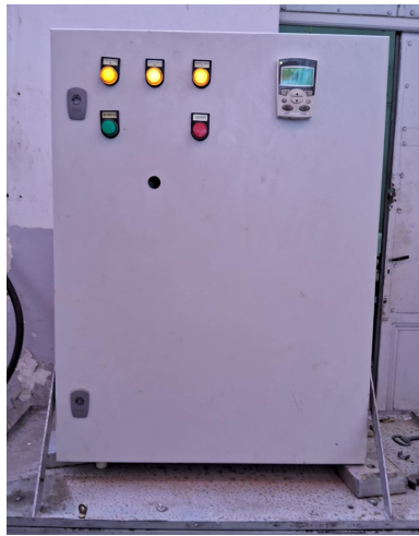
FIGURE 4.5 – Main control panel with integrated Variable Frequency Drive (VFD) for fan speed regulation.
