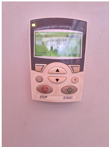
FIGURE 4.6 – VFD digital interface for controlling and monitoring the fan motor.
