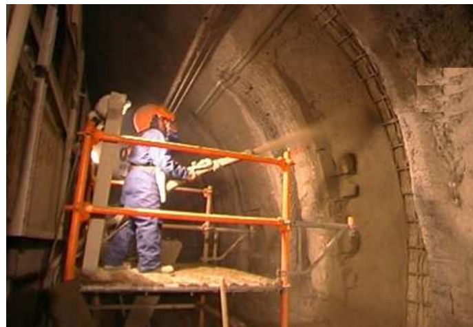
Figure III.8 : Béton projeté [12]
