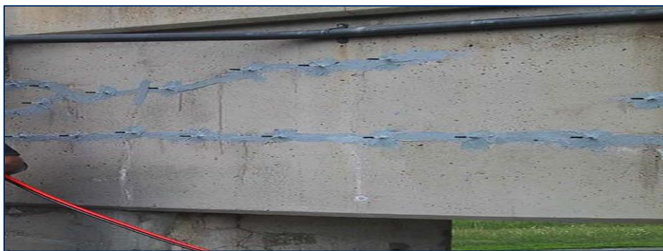
Figure IV.6. Injection des fissures
