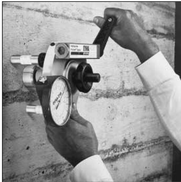
Figure III.10. Essai d'arrachement in situ
