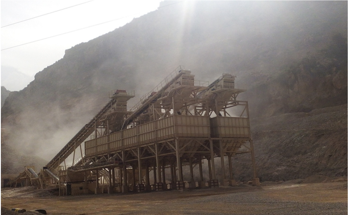
Figure VII.2 : station de concassage secondaire
