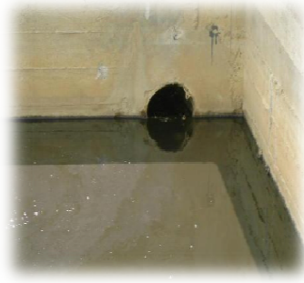
Figure 23: Canal d'évacuation de lixiviats.
