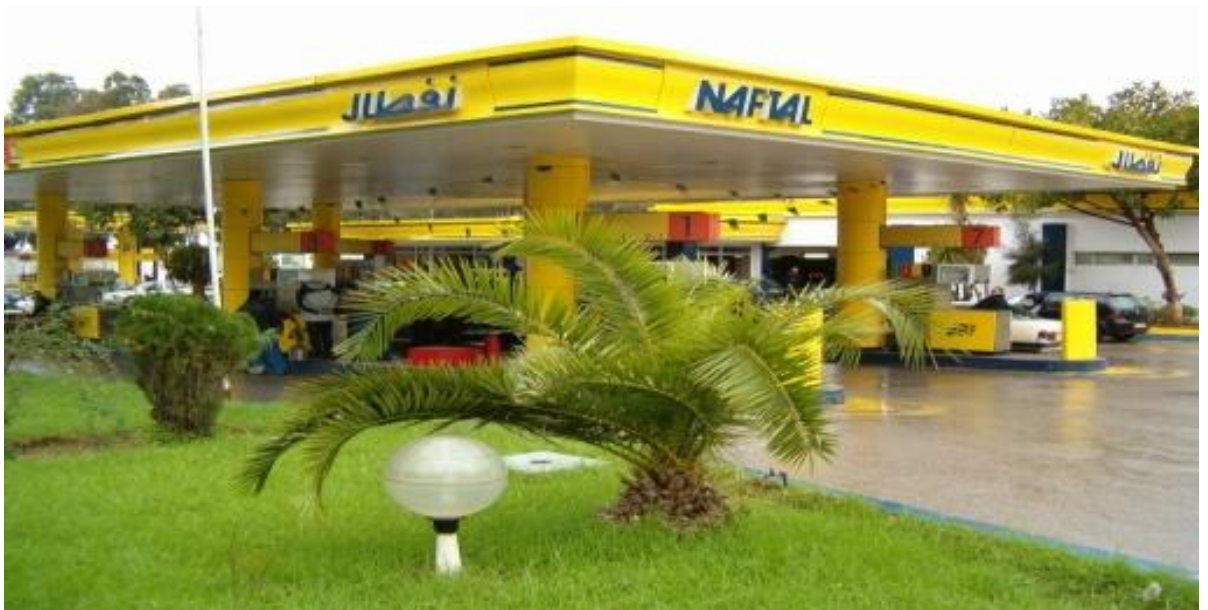
Figure I.1. Station de distribution
