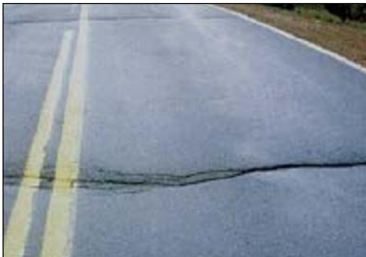
Figure I.7. Fissure transversale
