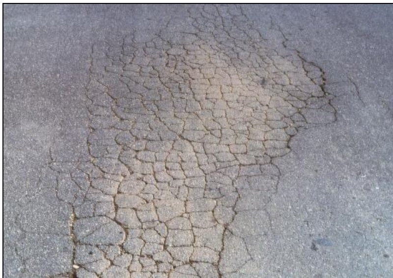
Figure I.9. Fissures polygonales
