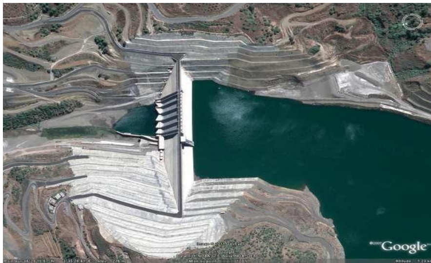
Figure II.4: Barrage de Koudiat Acerdoune (Google Earth, s. d.)
