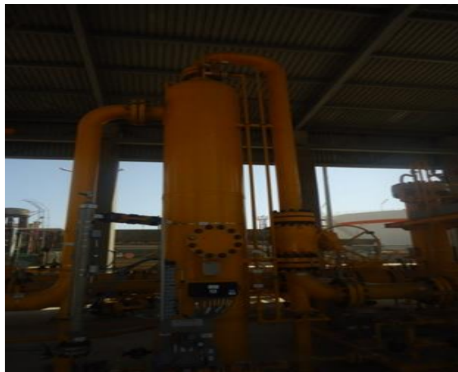
Figure 2.1 : Filtre cyclone
