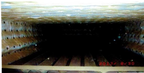
Figure 2.17 - Inspection de zone de convection
