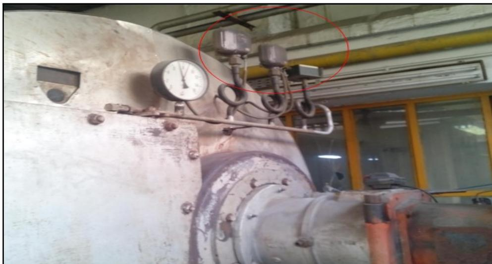
FIGURE 2.15 – Pressostats de la chaudière[Source exclusive]
