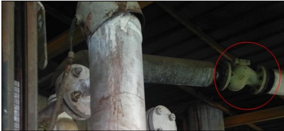
FIGURE 2.14 – Clapet anti-retour de la chaudière[Source exclusive]
