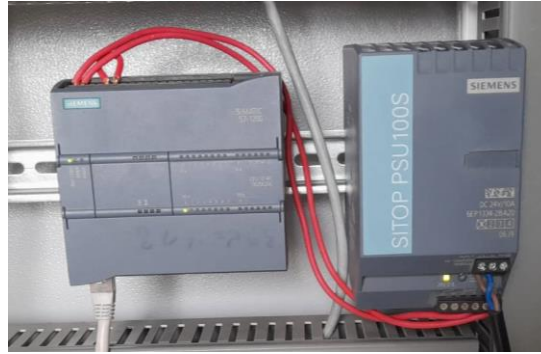
Figure 4.24 : Installation de l'automate S7 1200
