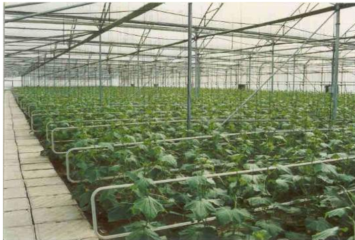
Figure 2.10: Hot water distribution system.[29]
