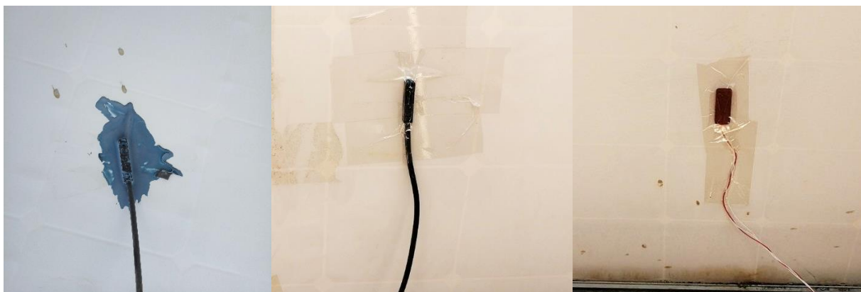
Figure 2.8 Three PT100 surface Sensors mounted to the back of modules.
