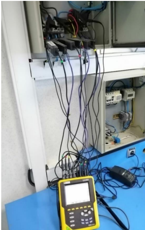
Figure 2.75 C.A 8336 installed on PCC.
