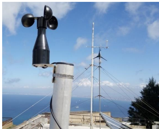
Figure 2.7 Wind velocity Anemometer.
