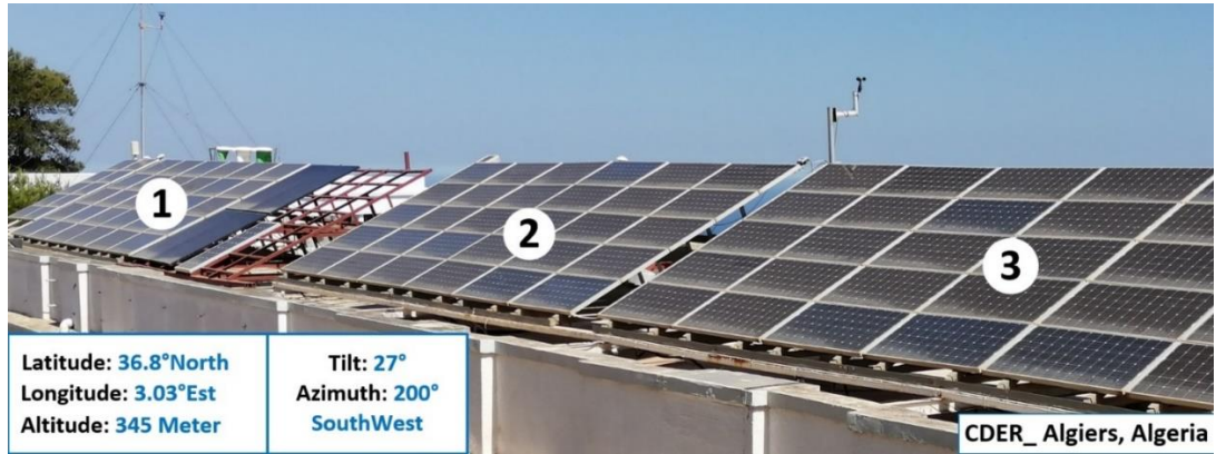
Figure 2.1 Picture of PV Array of the GCPV system on the top-roof at CDER.
