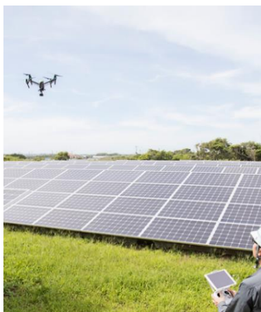
(b) Drone-mounted electroluminescence & thermal infrared imaging of PV arrays
