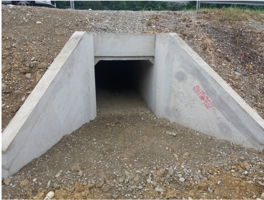
FIGURE I.4 – Photo d'un Dalot [4]
