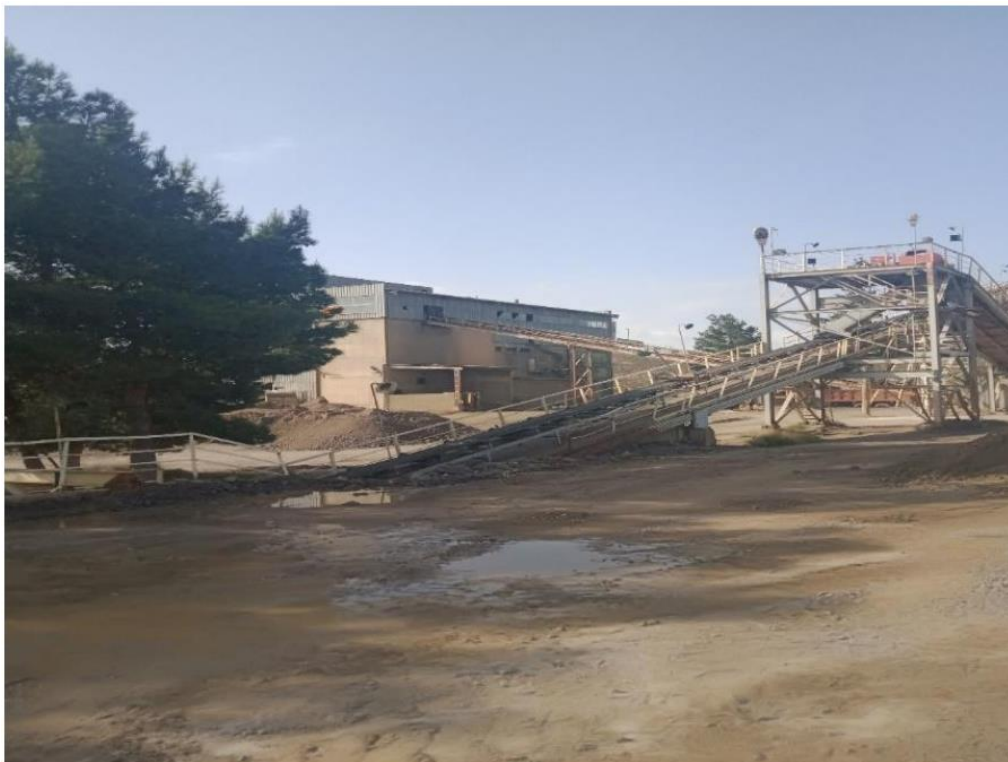
Figure 6: Usine de traitement complexe kherzet youcef (AKACHE Aymen ; BEDGHIOU Kaouther, 2021)
