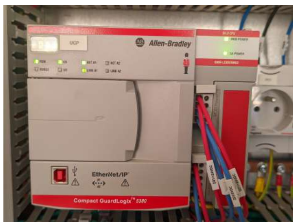
FIGURE 2.16 – PLC Compact GuardLogix 5380
