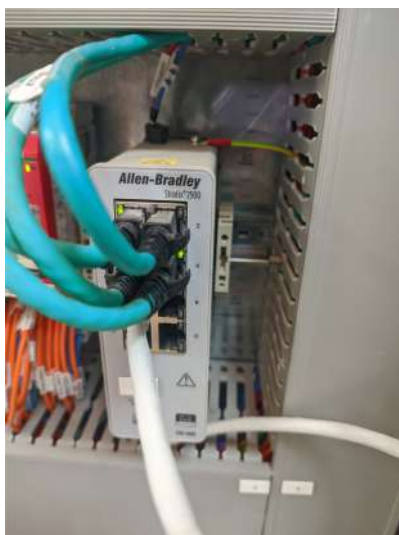
FIGURE 2.15 – SWITCH Ethernet/IP
