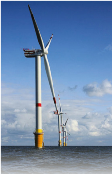
(a) Horizontal-axis wind turbine
