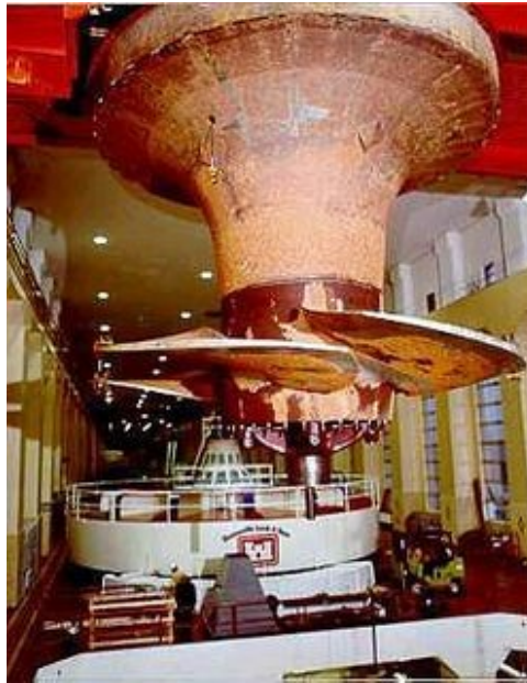
Figure I.4: Turbine de Kaplan [33]
