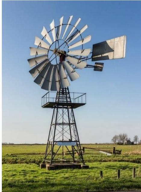
**Figure 1.1** Multi-blade wind pump.
