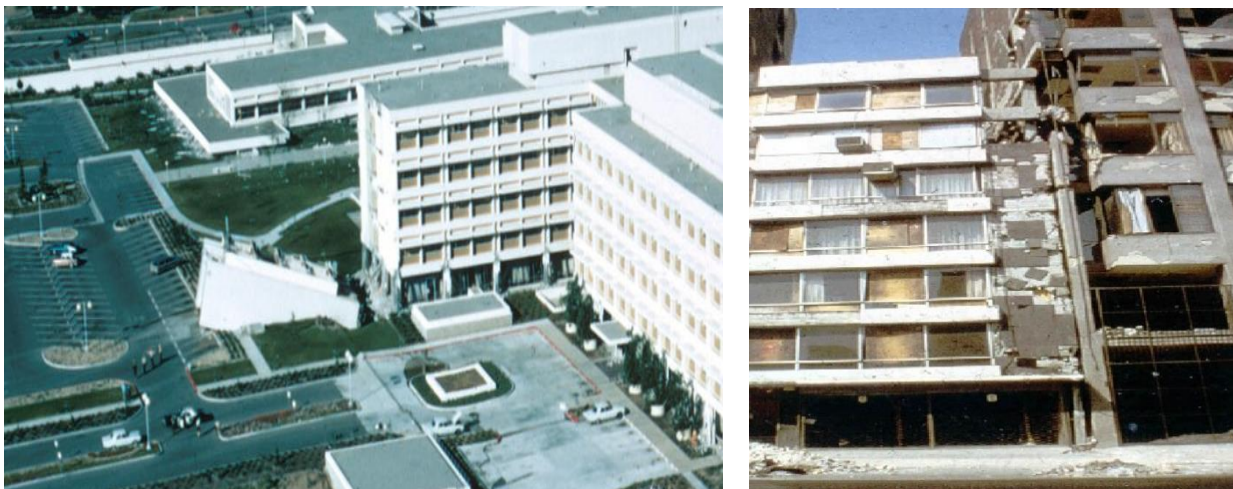
Figure VII-1: Examples of structural damage caused by pounding
