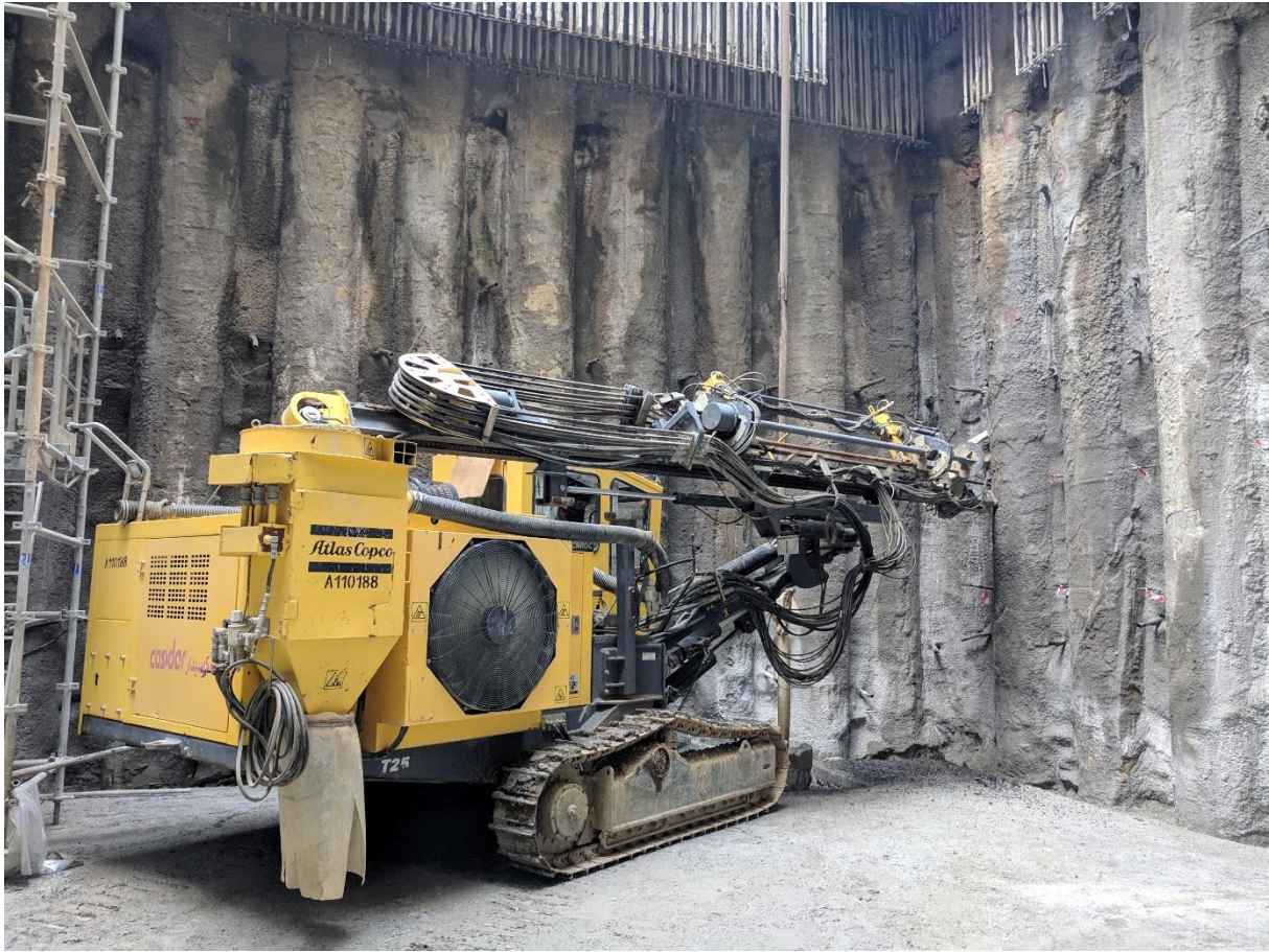
Figure 6.13- Chariot de forage ATLAS COPCO A110188
