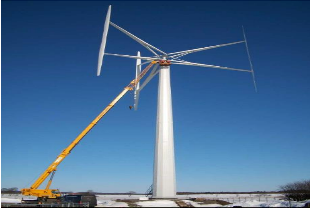
Figure 1-9: Eolienne verticale (3 pales, 200 kW, Falkenberg, Sweden) [4]
